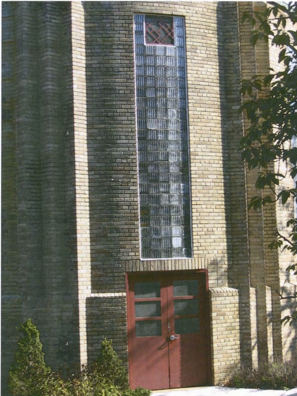
Illustration 4: Detail of glass block window and door on west side (DC Historic Preservation Office).
