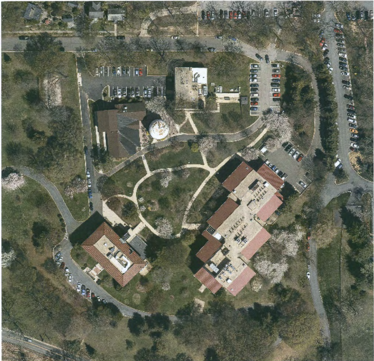
Map 2: Aerial photograph of the Carnegie Institution Broach Branch Road Complex. The Atomic Physics Observatory is the round white structure at the center of the complex.
