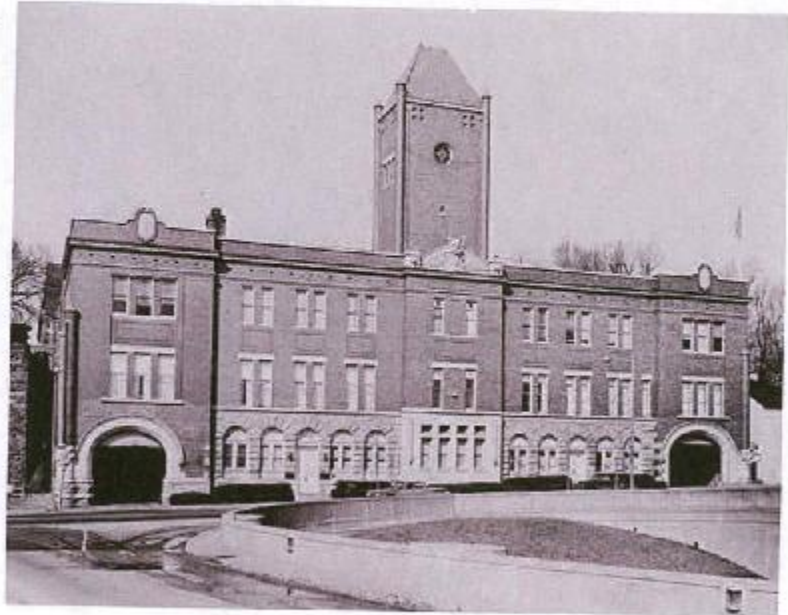
Photo 1. Historic American Survey Marc Blair Photographer, summer 1966 South (front) Façade. Historic American Building Survey (HABS No. DC-125), "Capital Traction Union Station," Library of Congress, Prints and Photographs Division.
