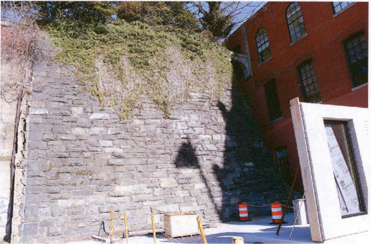
Image 7 of 19. Stone-faced Retaining Wall, looking northeast.
