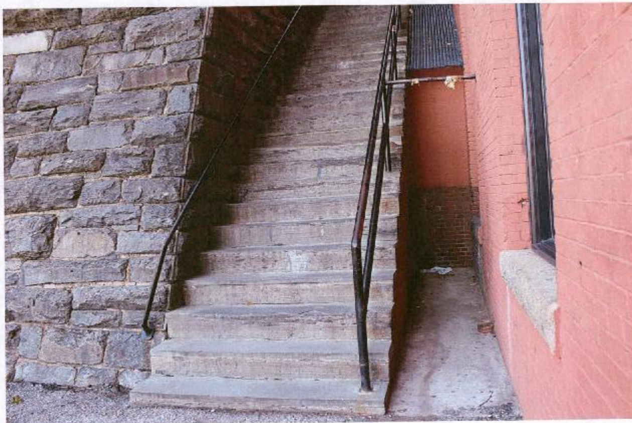
Image 6 of 19. Base of Exorcist Steps, looking northwest.
