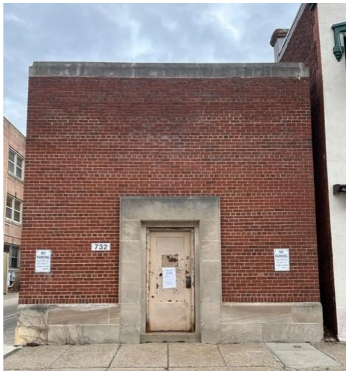
732 7 th Street SE as seen from 7 th Street
