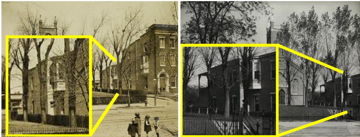
The former rear addition as it appeared in photographs from the early twentieth century. The image within each yellow square is a zoomed in portion from the photographs. (Images from the DC Public Library).
