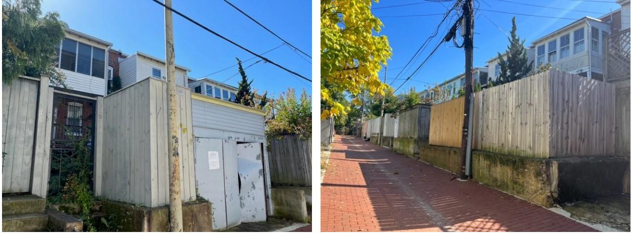
Views of the rear of 616 Lexington and adjacent properties from the alley
