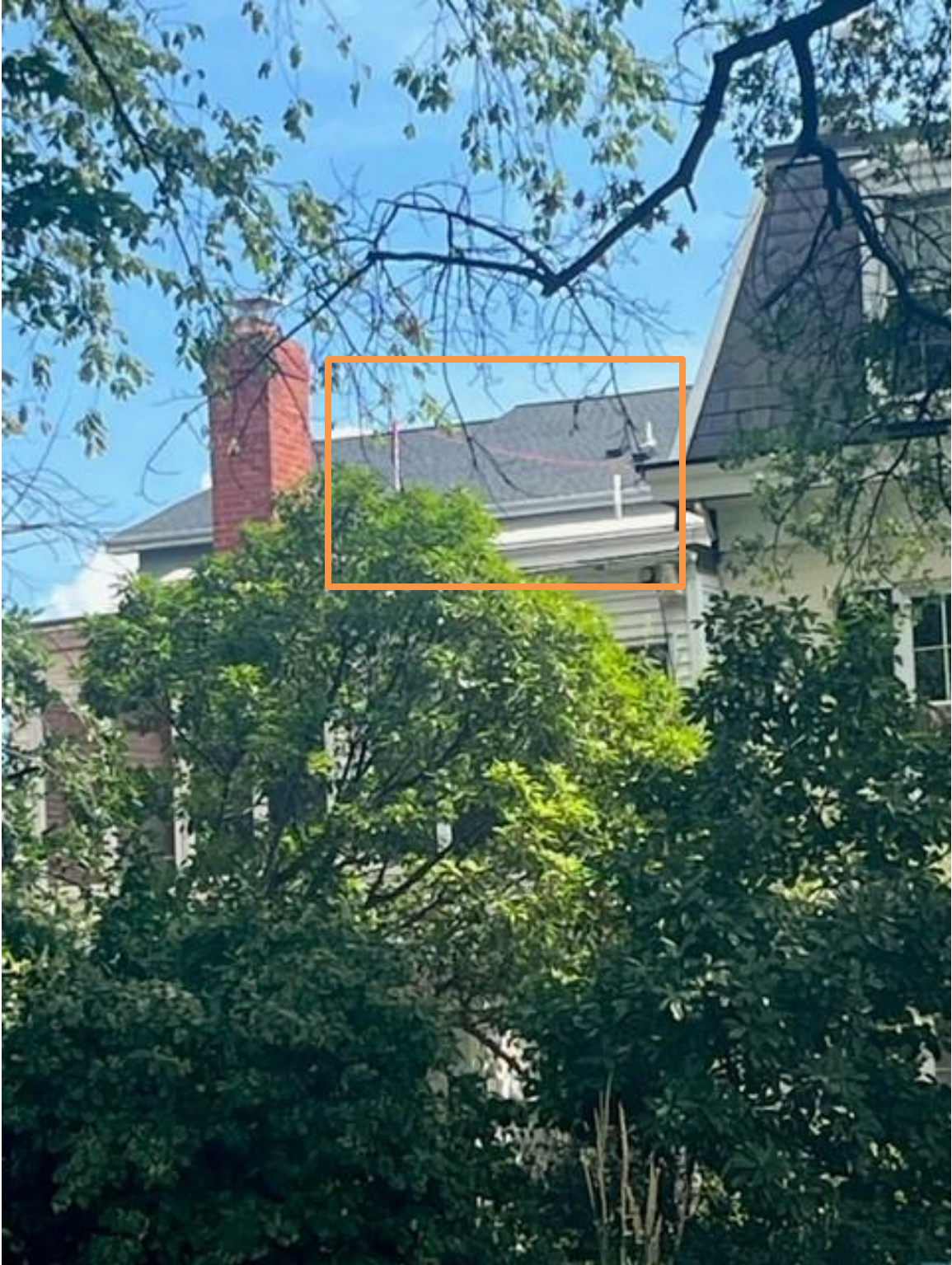
Mock-up of rear addition front wall visible from E Street
