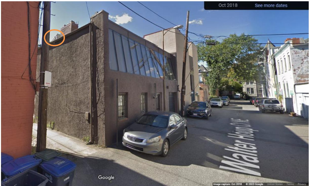
View of 5 Walter Houp Court from alley, shed structure visible and circled
