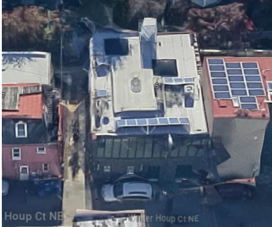
Google aerial view of roof of 5 Walter Houp Court NE
