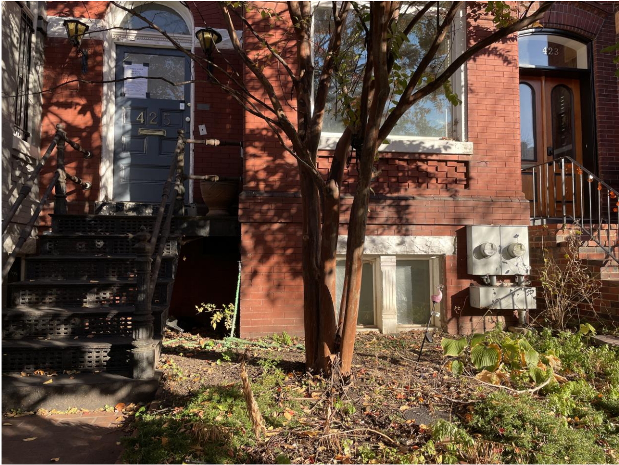
Front of the house depicting the existing cellar window.
