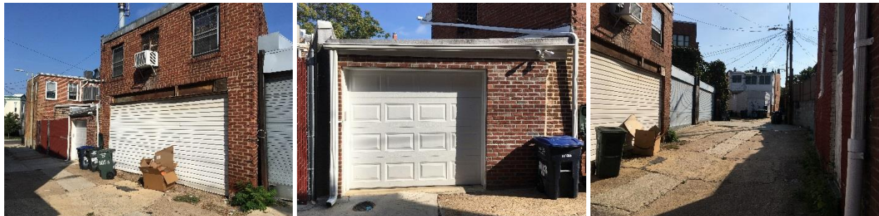
Contextual views of the rear of property from the alley
