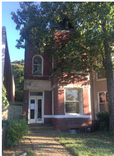
Front elevation of 715 North Carolina Avenue, SE
