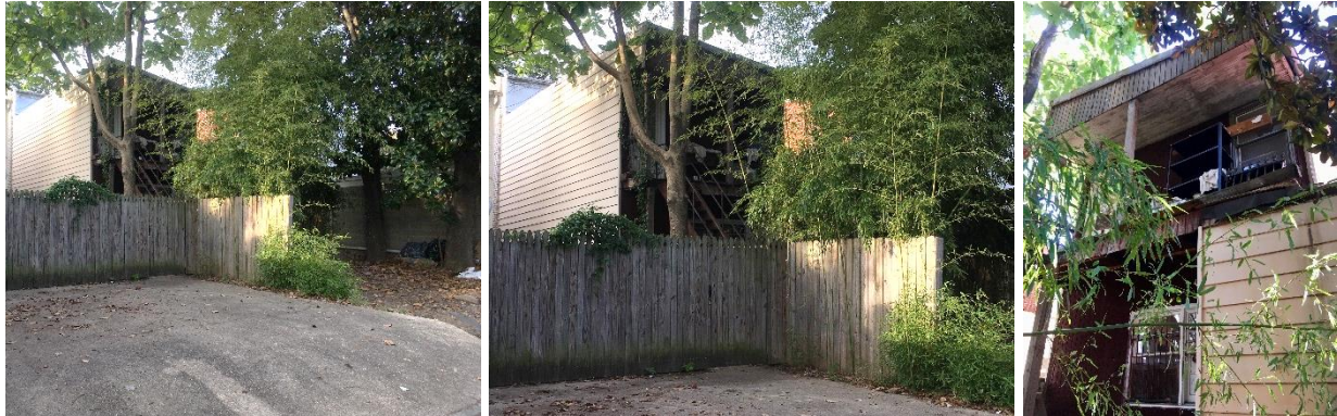
Views of the rear of property from the alley
