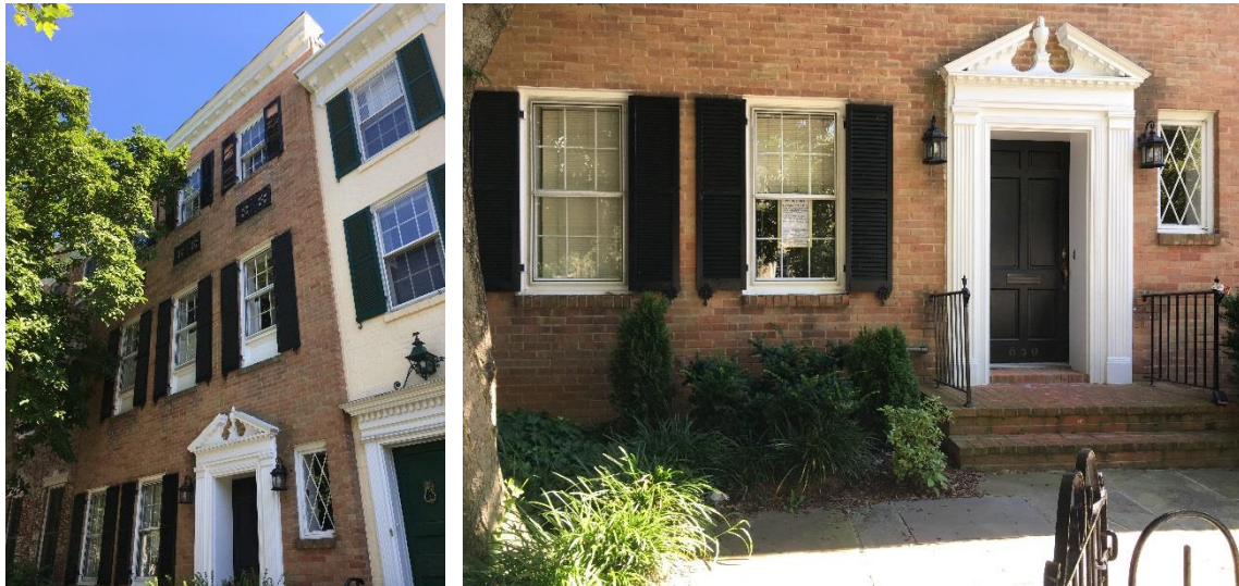
The front elevation of 639 E Street, SE
