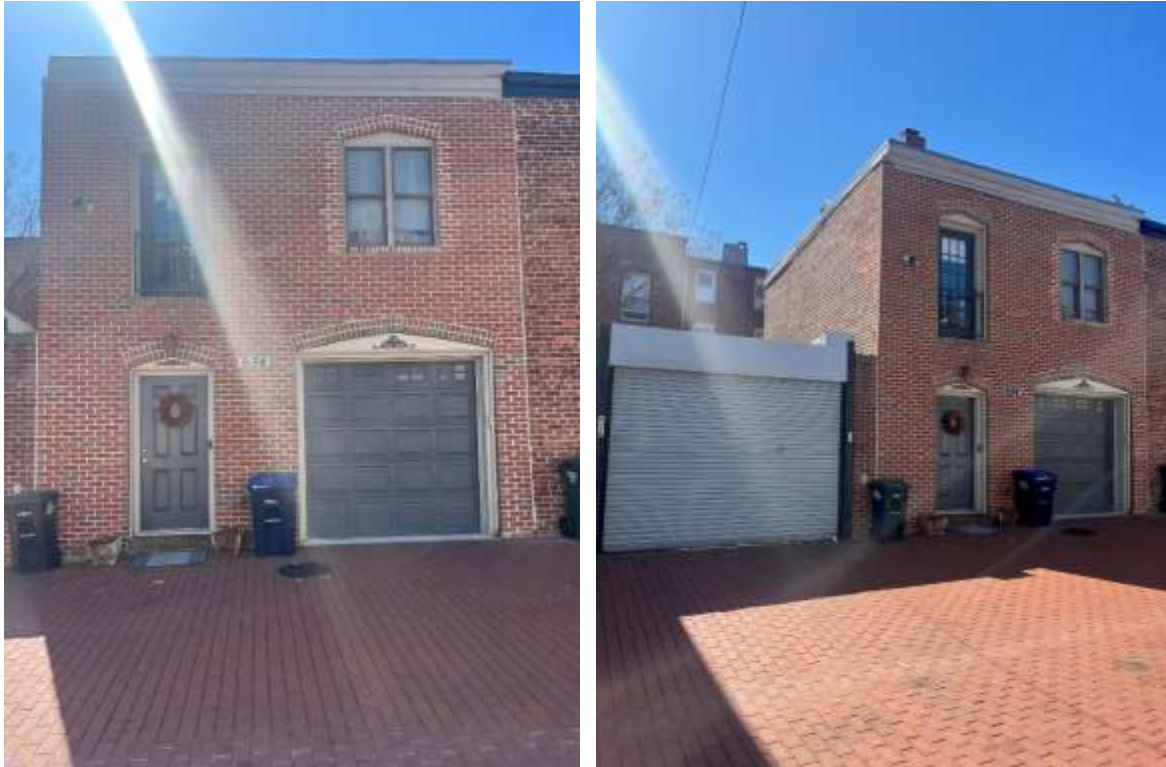
Views of the existing two-story carriage house and rear of house from the alley
