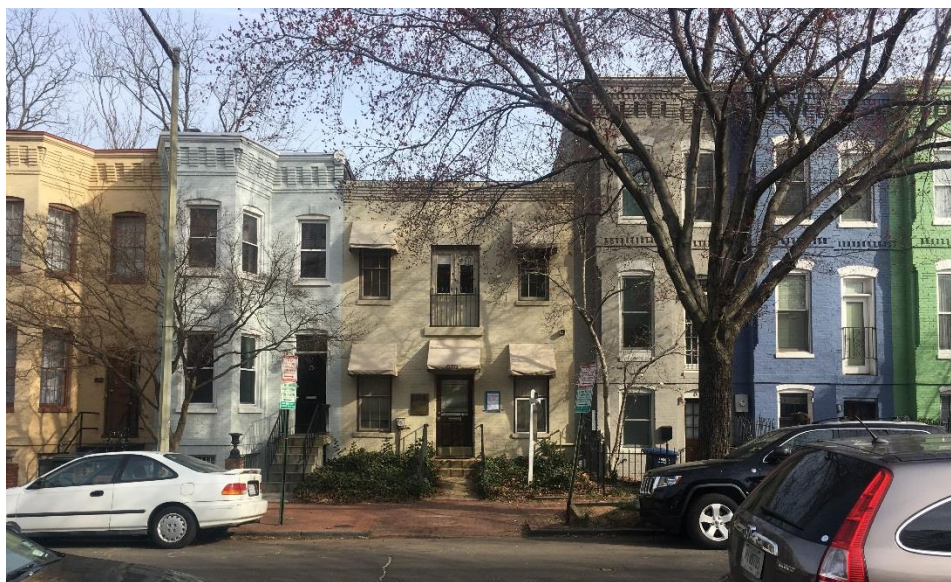
Across the street view of the property
