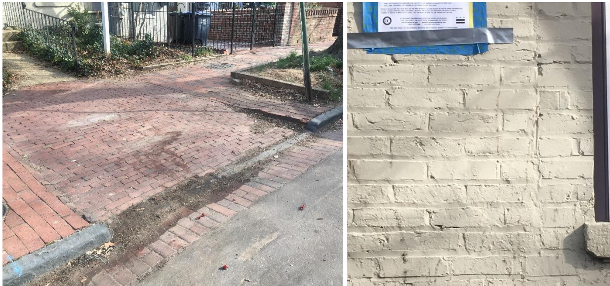
The existing curb cut and an example of alteration to the brick on the facade
