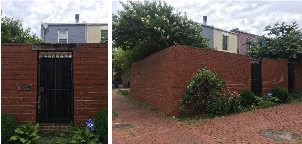
Contextual views of the property and row from the rear
