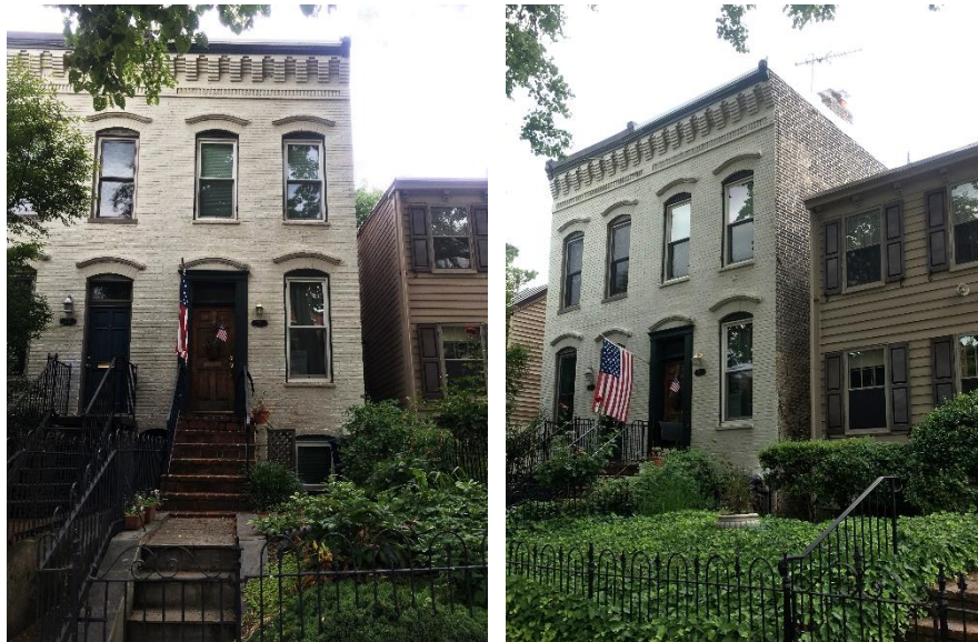
The front elevation of 511 5 th Street, SE
