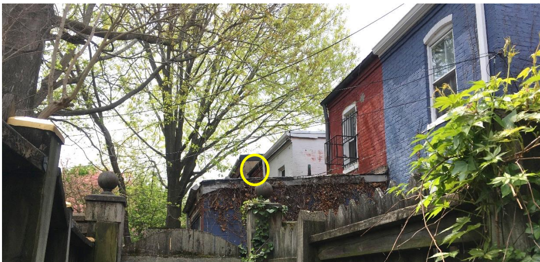
Limited accessibility to rear views of the property, corner of 429 roofline circled
