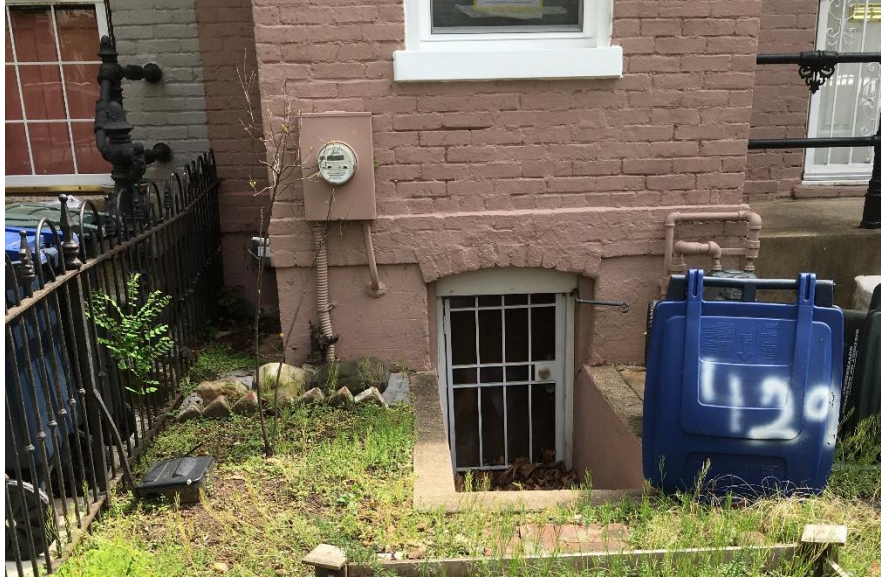
Existing front basement window well as visible from the sidewalk
