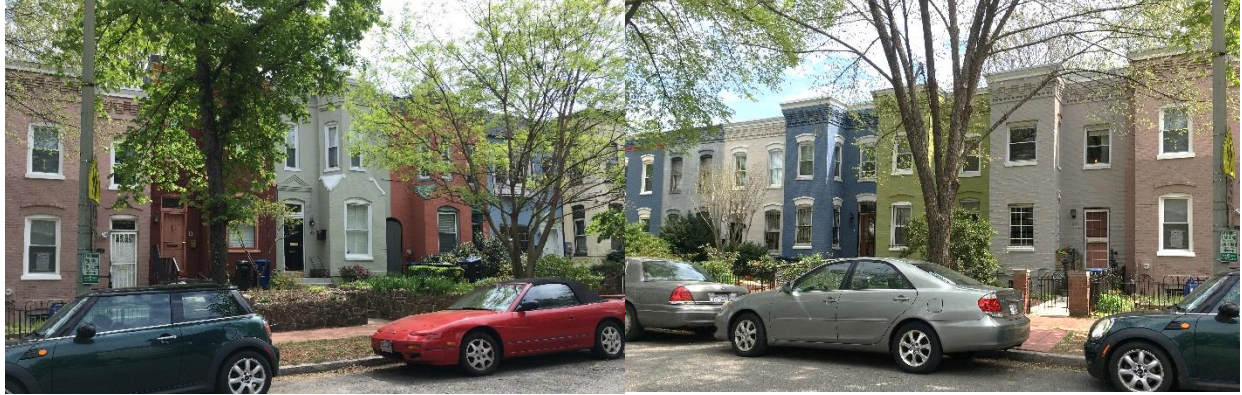
Contextual views of the property
