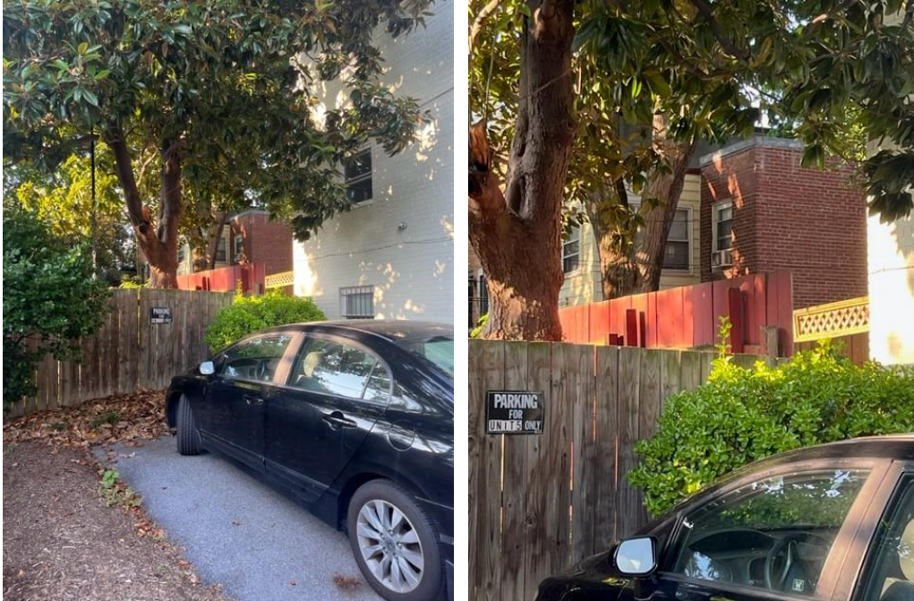
Views towards the rear of 323 10 th St SE from nearby alley
