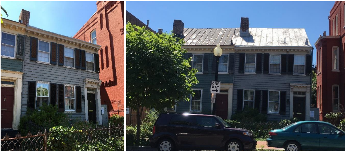
The front elevation of 321 6 th Street, SE
