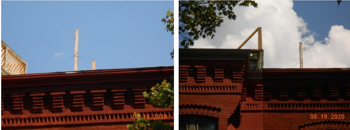
Close-up views of lumber mock-up
