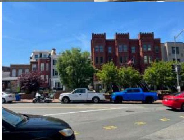
Views of 227-239 Massachusetts Avenue NE from the opposite side of the street.
