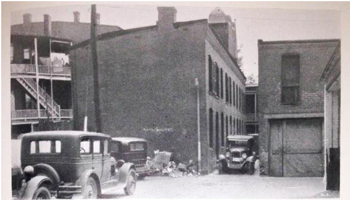
PROJECT NO. 1. This nest of five alley houses, facing a brick wall in Rupperts Court, was the first purchase of the Authority. The houses were crowded into the interior of a square. The principal street boundary of the square is a commercial artery. Other buildings in this alley were used for commercial purposes
