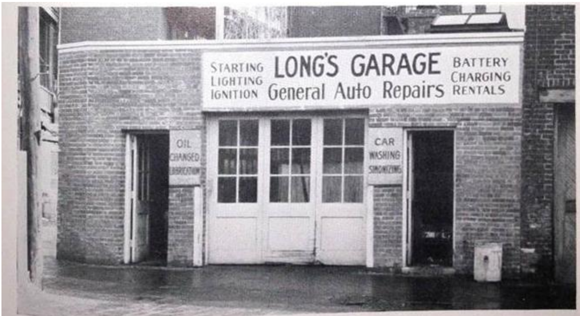
WHERE ALLEY HOUSES STOOD. Constructed by the Authority on the site of Rupperts Court alley houses, this repair shop completes commercial development of the alley. The Authority has leased the shop to a private tenant
