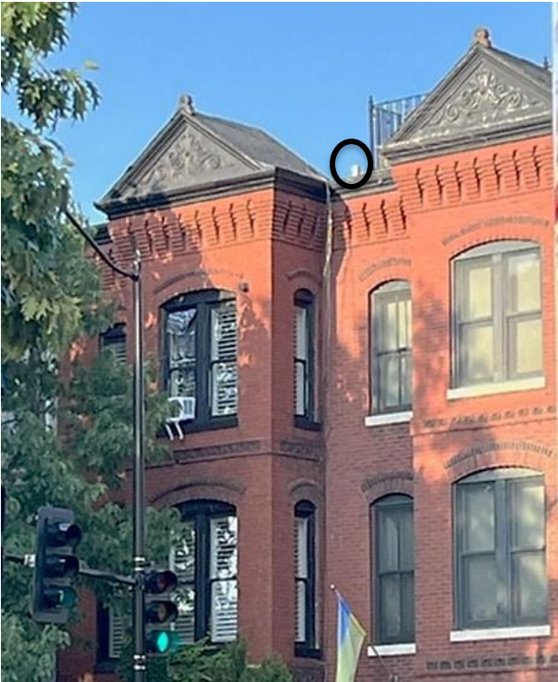
510 9 th Street viewed from the West; flag test visible over the roof
