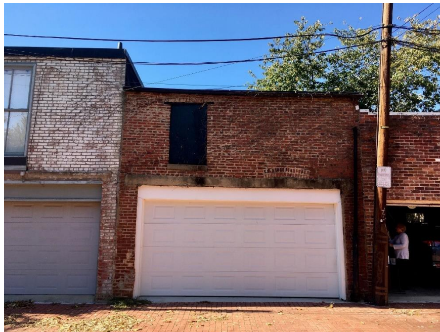
Existing 1877 stable building at 152 11 th St SE
