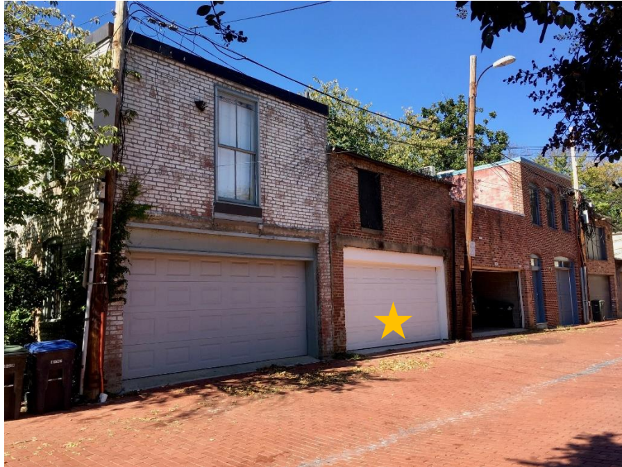
View of the stable building (with star) and adjacent garages
