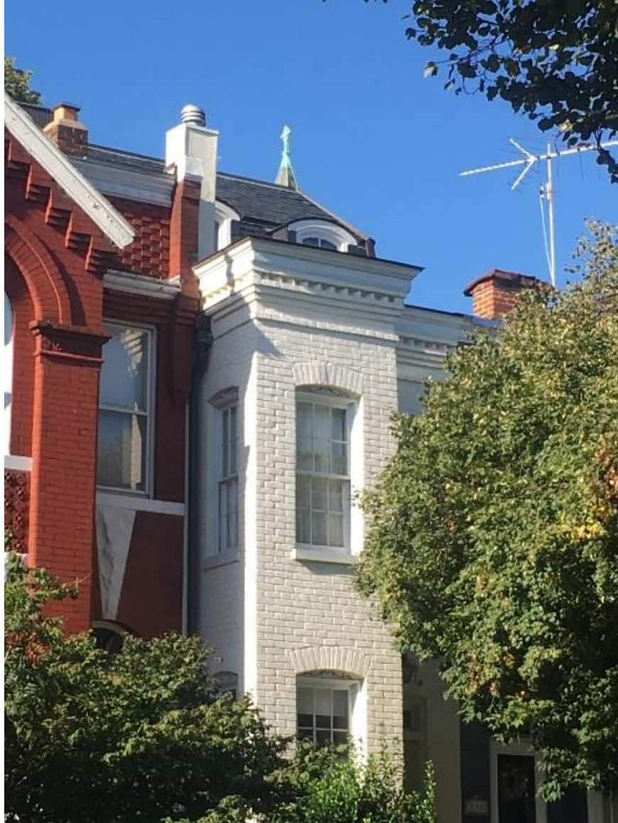
Visible rooftop addition at 140 D Street SE
