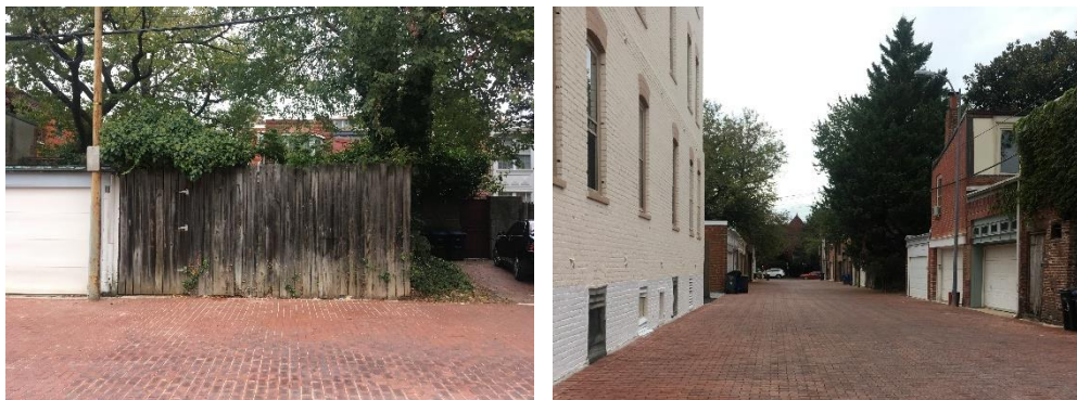
Views of the rear of property from the alley
