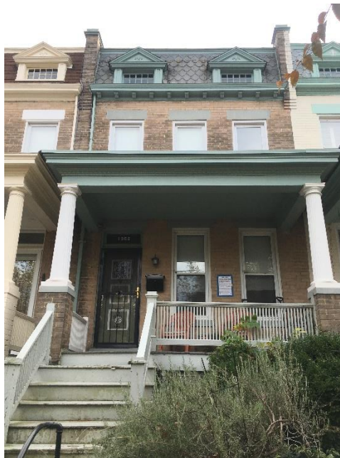
Front elevation of 1355 A St NE
