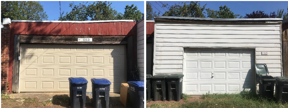
The alley-facing elevations of the garages at 1363 and 1365 A Street, NE
