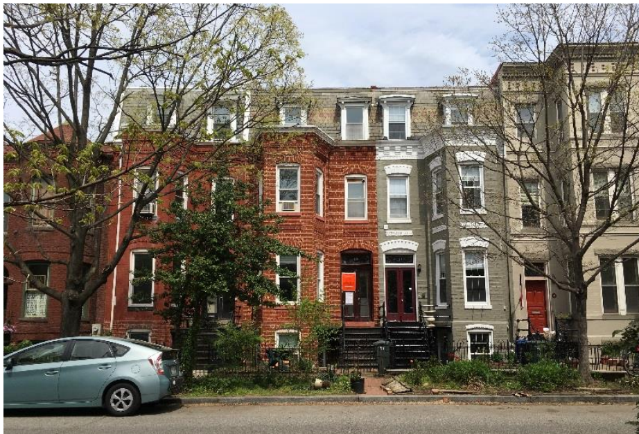
View of 414 from across Constitution Avenue
