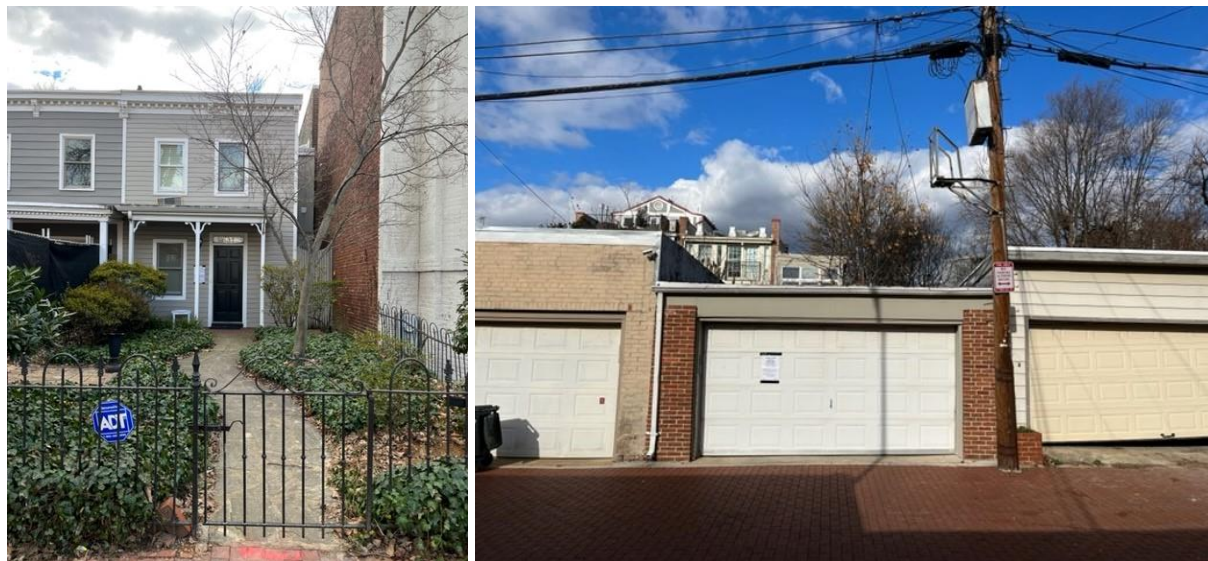
637 A St SE seen from the front (left) and rear (right)
