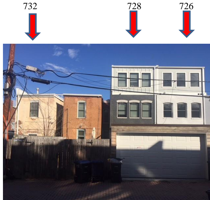
Figure 1: Existing conditions at the rear of the property
