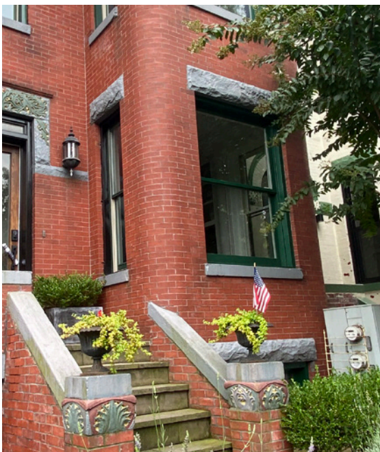
Double wide double hung sash windows
