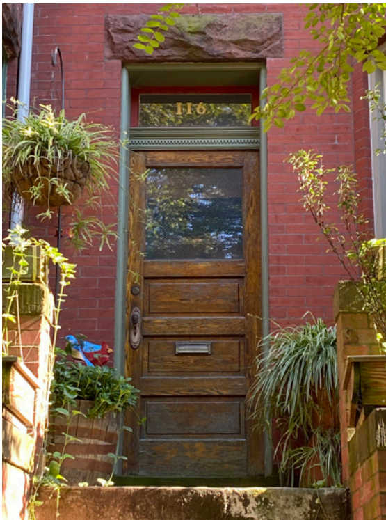
Original wood panel door with glazing
