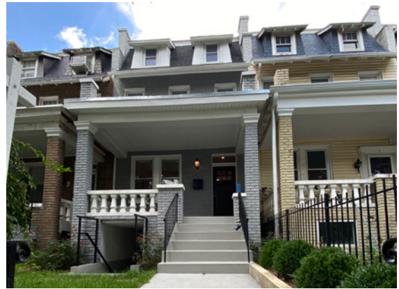
Maintained porch details with masonry piers and original cast stone railings
