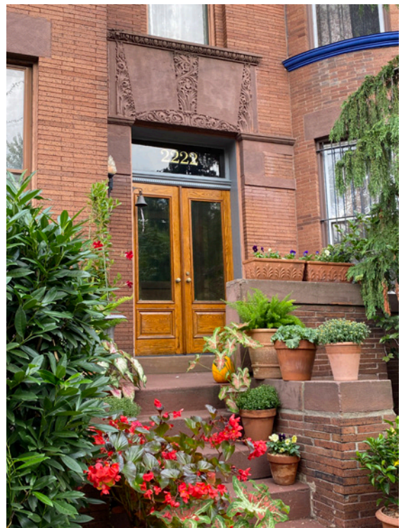
Double door fits in original opening
