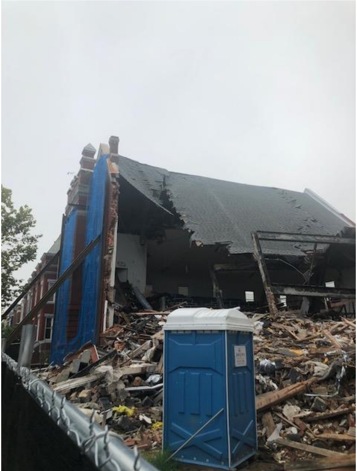
150 S Street NW, unsupported roof (September 16, 2018)
