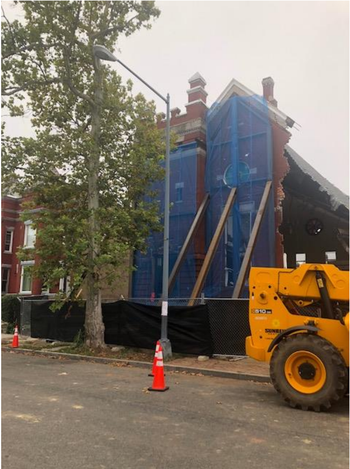
150 S Street NW, stabilization of façade (September 16, 2018)
