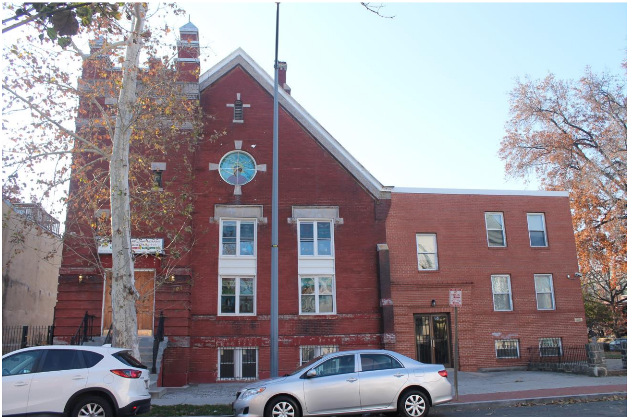
150 S Street NW, prior to unauthorized demolition
