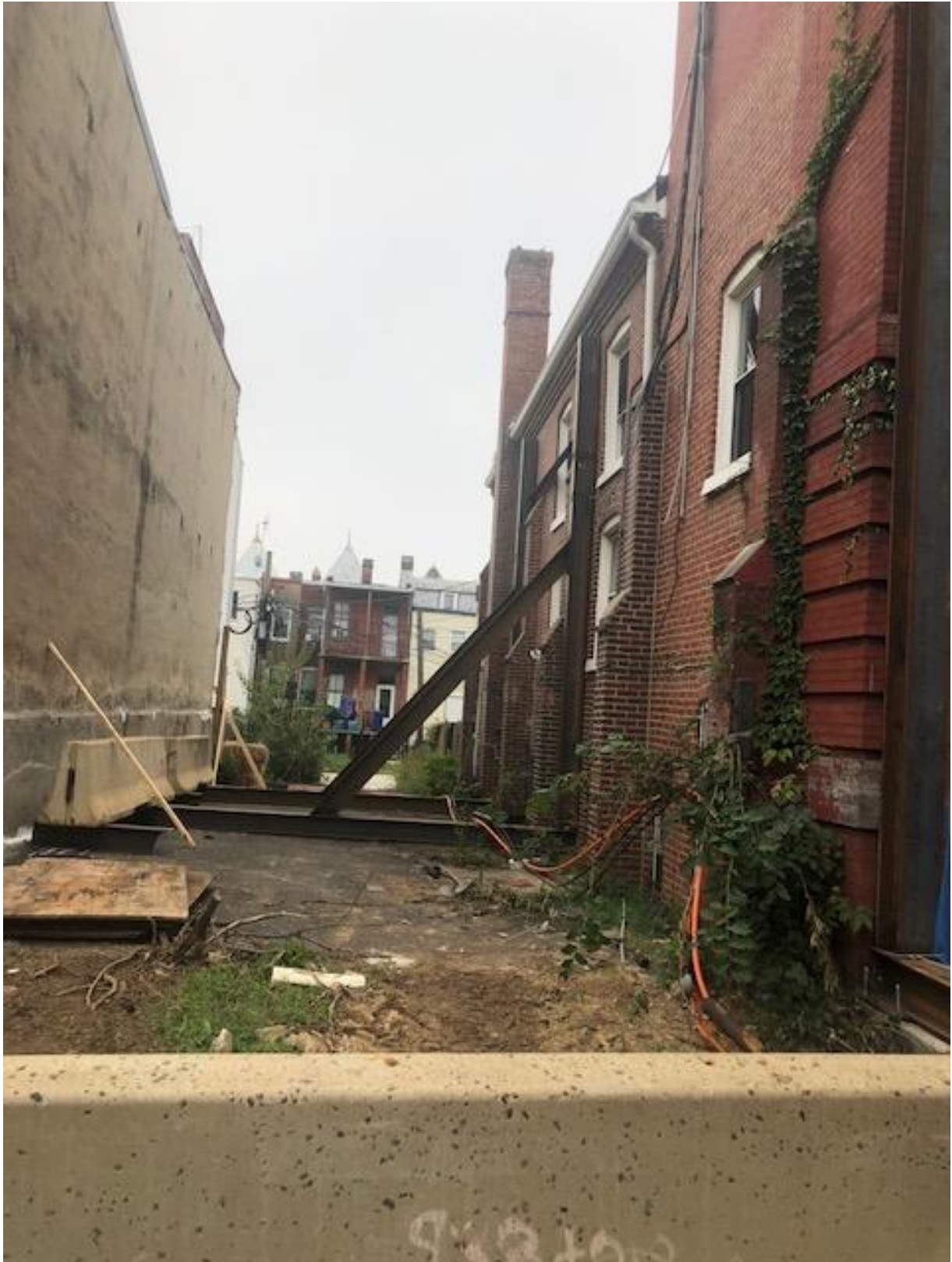
150 S Street NW, stabilized side elevation (September 16, 2018)
