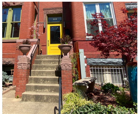
Addition of simple metal handrails
