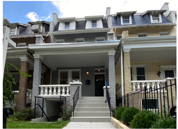
Maintained porch details with masonry piers and original wood railings
