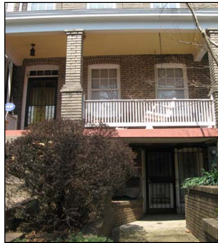
Excavating front yards and removing porch piers for at-grade access to the basement is not appropriate.
