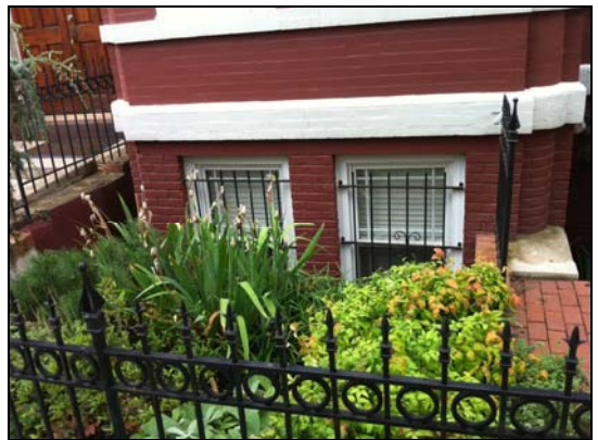
A small window well, screened with landscaping, may allow basement windows to be lowered for additional light.
