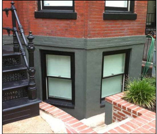
This new basement areaway was designed to replicate original areaways on similar houses in the area.
