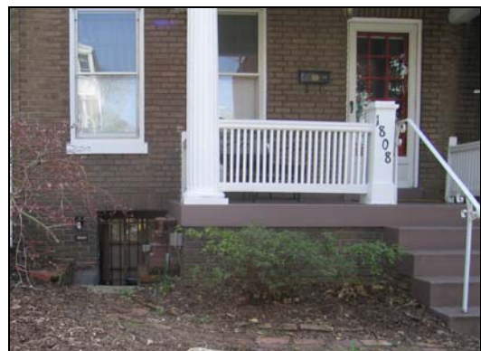
On a partial-width front porch house, locating the basement entrance at the front wall of the house or on the side of the porch can minimize its visual impact. The new door is secondary to the porch and main entrance.
