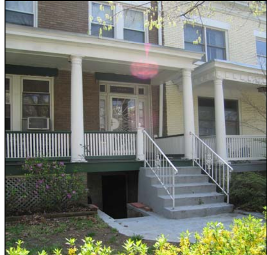
This front basement entrance only resulted in the removal of a portion of the lattice skirt and preserved the character defining features of the porch.
