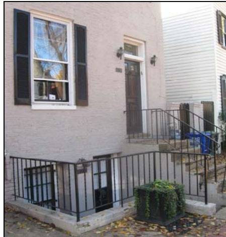
This large areaway results in the house sitting in a pit, exposes large portions of the structure's foundation walls, and changes the relationship of the house to the street.
