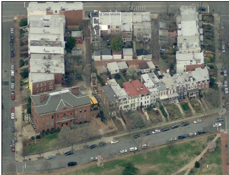
View of the subject block looking north across South Carolina Avenue
