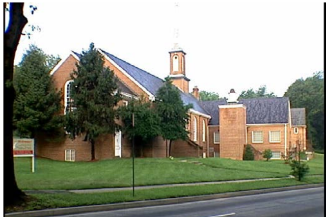
1600 Taylor Street NE, 1949 District of Columbia Office of Planning 2004
