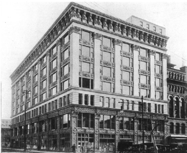
Woodward and Lothrop Building, built 1902 G Street between 10 th and 11 th Streets, N.W. Library of Congress Prints and Photographs Division, HAB-DC 546-1
