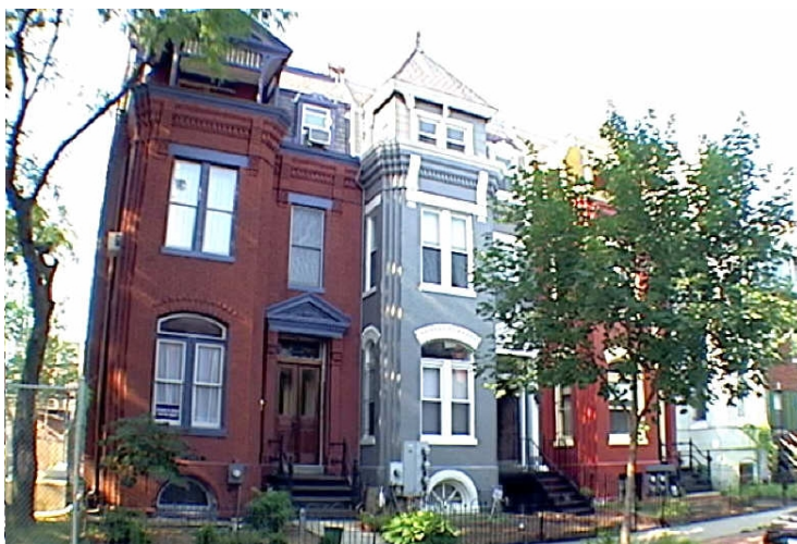
Rowhouses (Greater U Street), 914-918 S Street, NW D.C. Office of Planning, PropertyQuest, 2004
