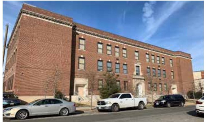
BUNDY SCHOOL, 429 O STREET NW
