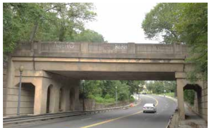
B&O RAILROAD BRIDGE OVER MONTANA AVENUE NE
