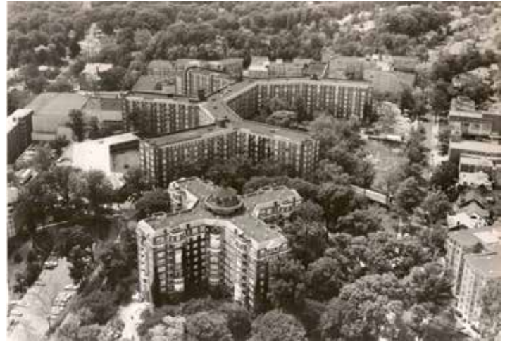
WARDMAN PARK ANNEX, SHOWING DEMOLISHED HOTEL BEHIND
