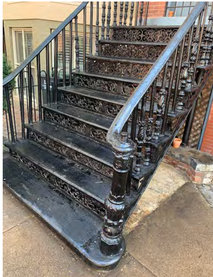
RESTORED AND REPAIRED CAST IRON RAILING
