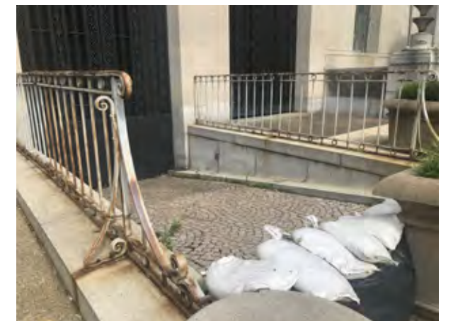
VEHICULAR RAMP AT THE ROBERT F. KENNEDY BUILDING
