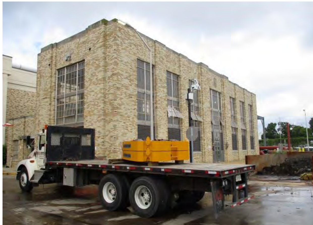
BLUE PLAINS FACILITY SURVEY - RAW WASTEWATER PUMP STATION #1
