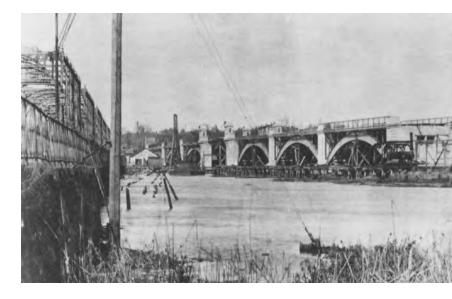
In 1874, after many years of wooden replacement bridges crossing the Anacostia at the Navy Yard, Congress authorized the construction of a wrought iron truss bridge (at left in photo). As the 1874-75 bridge become inadequate for motor and rail traffic, a new steel arch bridge, shown under construction in this 1908 photograph, was built to replace it. The present, twin-span Eleventh Street Bridge replaced these earlier bridges in 1965-70
