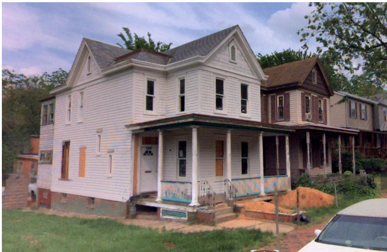
Gable-fronted houses on 25-foot-wide lots next door to 1350-1352 Valley Place SE.
