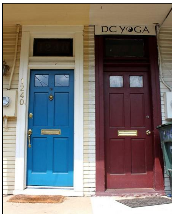
Historic wood doors in Anacostia generally had 4- or 5-paneled configurations and sometimes incorporated glazing on the upper panels.
