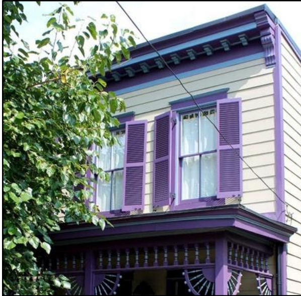
Compatible, operable louvered wood shutters
