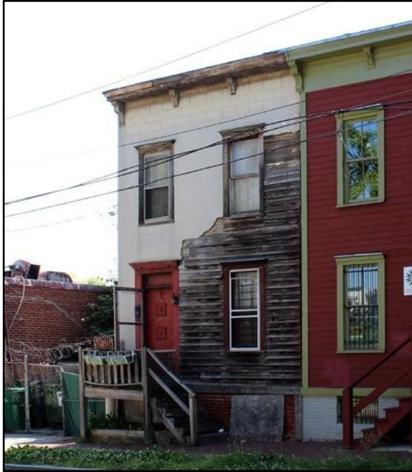
Here, stucco was applied directly atop the earlier cladding.
