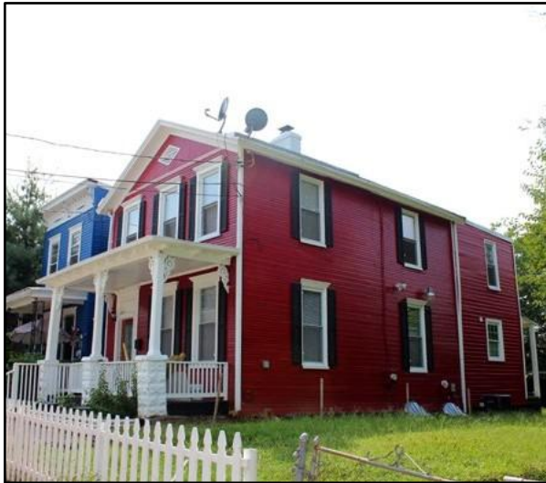
In this compatible rear addition, altering the profile of the siding, the roofline, and the window size allowed the addition to be clearly defined from the original building.
