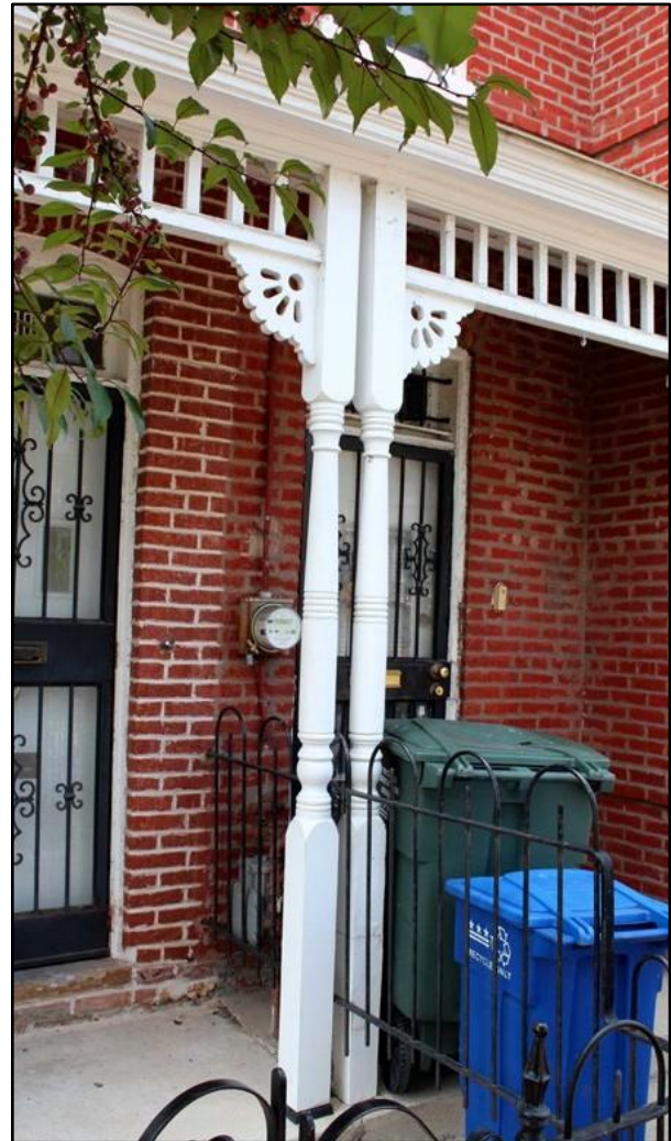
The elements on the left are modern replacements. They were replicated to match existing components on the adjoining house.
