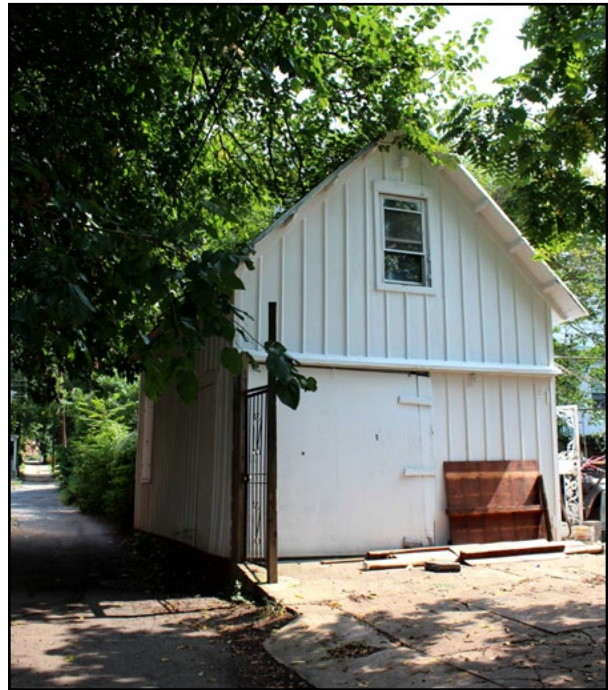
In this compatible rear addition, altering the profile of the siding, the roofline, and the window size allowed the addition to be clearly defined from the original building.
