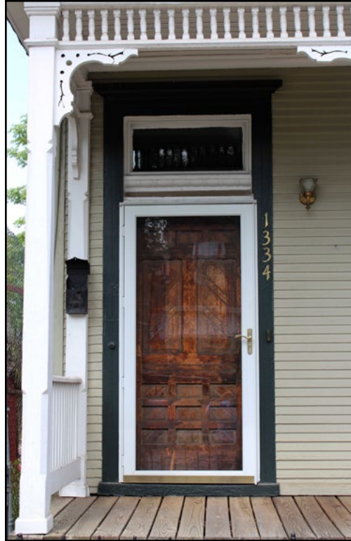
The addition of glazed storm doors allowed these original doors to be seen and protected and improves their energy efficiency.
