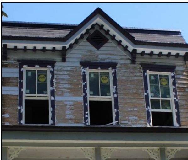
Windows here are being replaced to match their historic appearance and glazing pattern.
