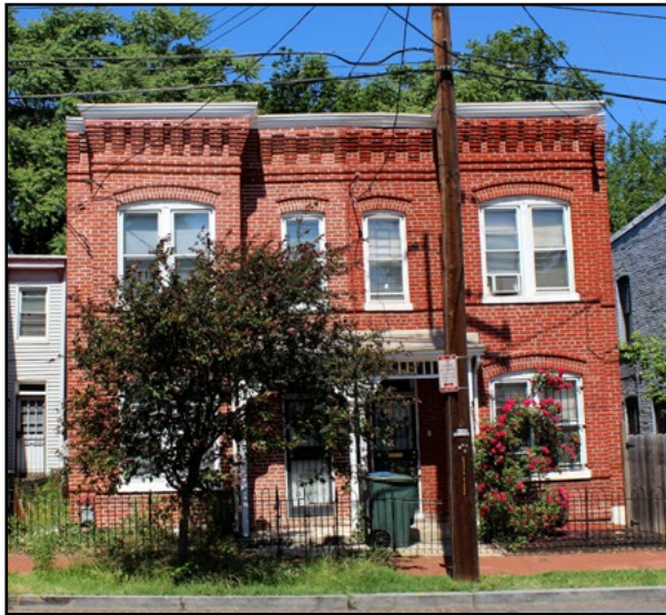
The house on the left was recently repointed. The mortar successfully reproduced the composition and color of the original.
