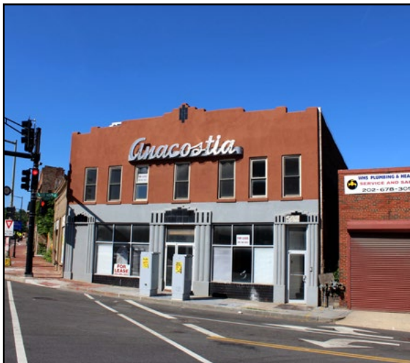
Commercial buildings in the Anacostia Historic District
