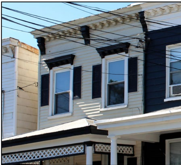
These incompatible, fixed vinyl shutters do not match the height or width of their corresponding windows.
