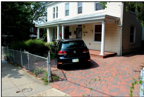
Parking spaces should never be located in the front yard. The extensive paving used to create this drive is not compatible with the character of the original landscape.
