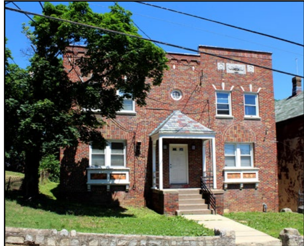
The façade of this small apartment building incorporated a mix of masonry materials and patterns.
