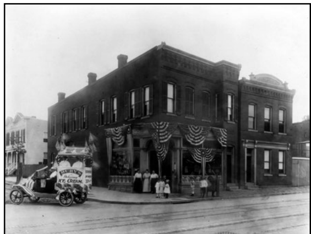
Commercial buildings on the 2200 block of Nichols (now Martin Luther King, Jr.) Avenue, circa 1919 Library of Congress
