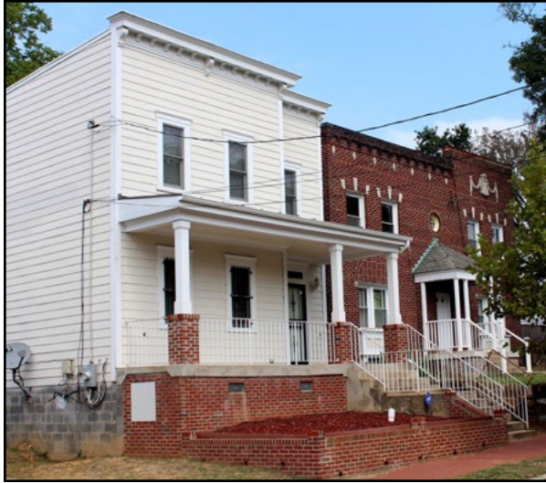
Fiber-cement siding was used on this new building.
