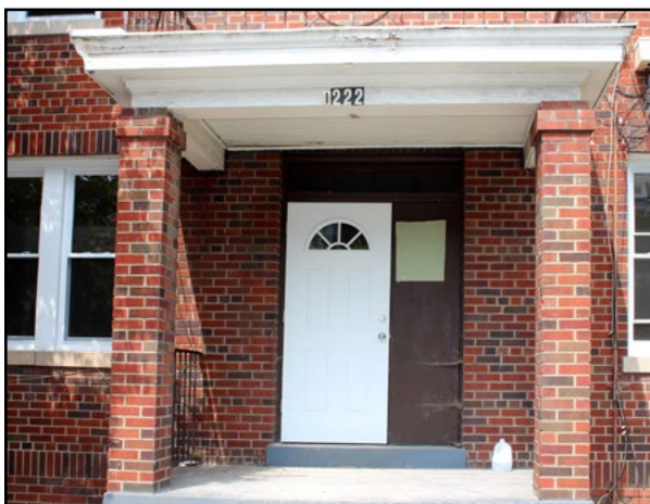
Fanlight-style doors are not appropriate replacements.
