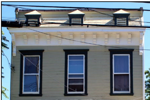
Decorative wood cornices or pent roofs were often used to embellish façades and conceal sloping roofs.
