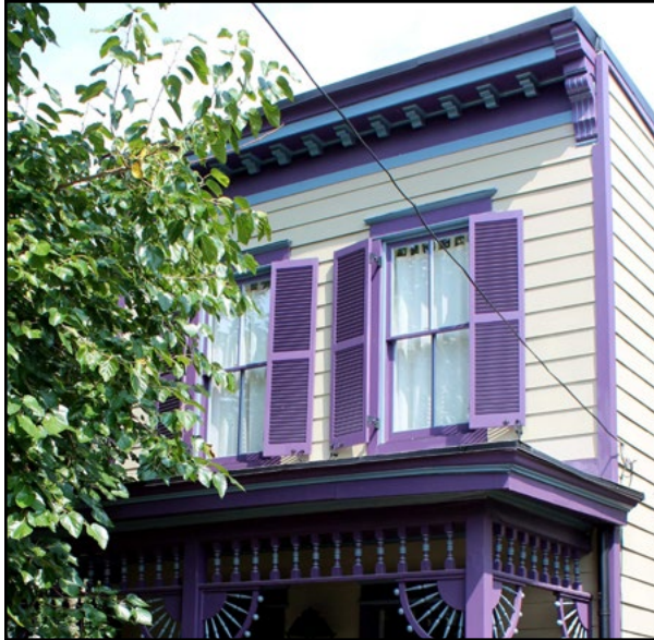
Compatible, operable louvered wood shutters
