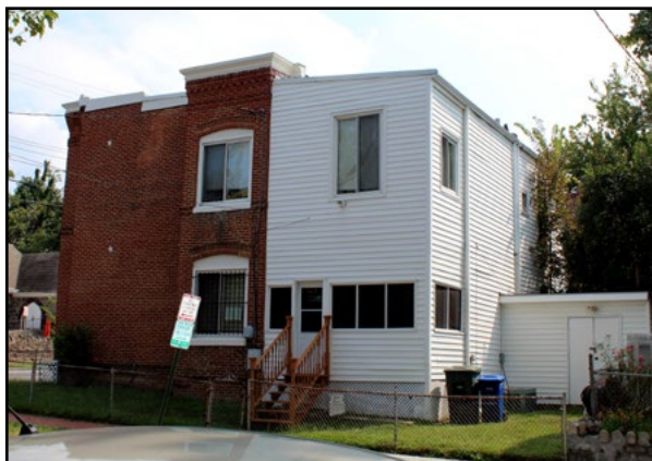
The prominence and projection of this incompatible addition visually competes with the original building. The addition's side wall should have been aligned with that of the house, set behind the bay.
