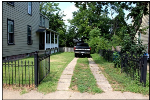
Gravel (above) or parallel tracks of concrete divided by turf (below) were common historically.
