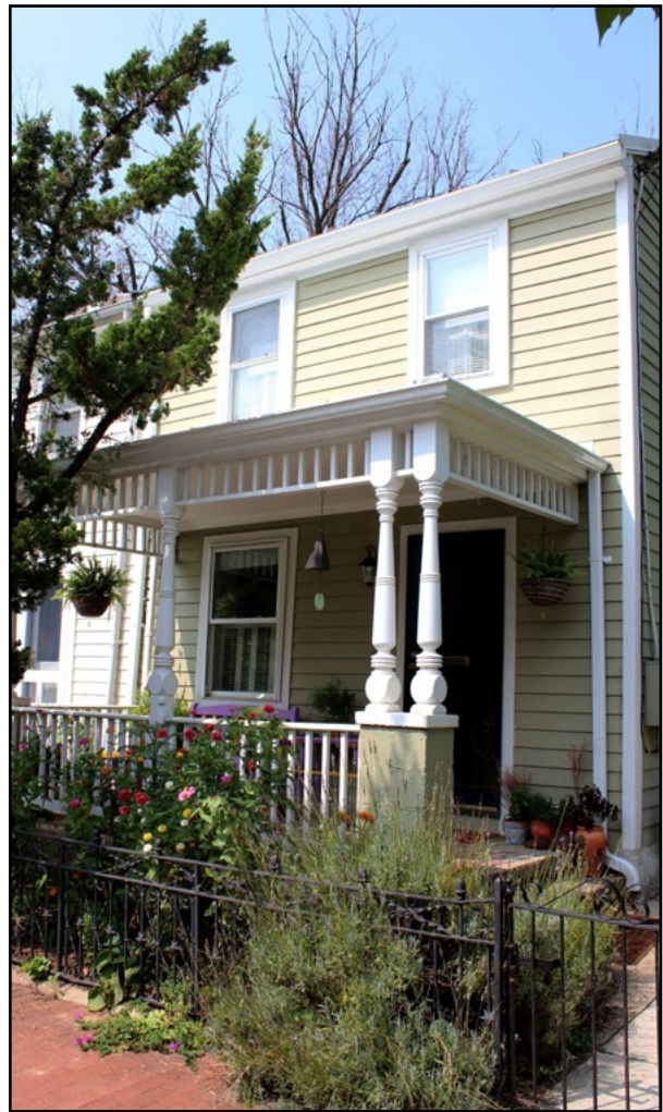
This porch of this house features a spindlework frieze, elaborately turned posts, and masonry piers.
