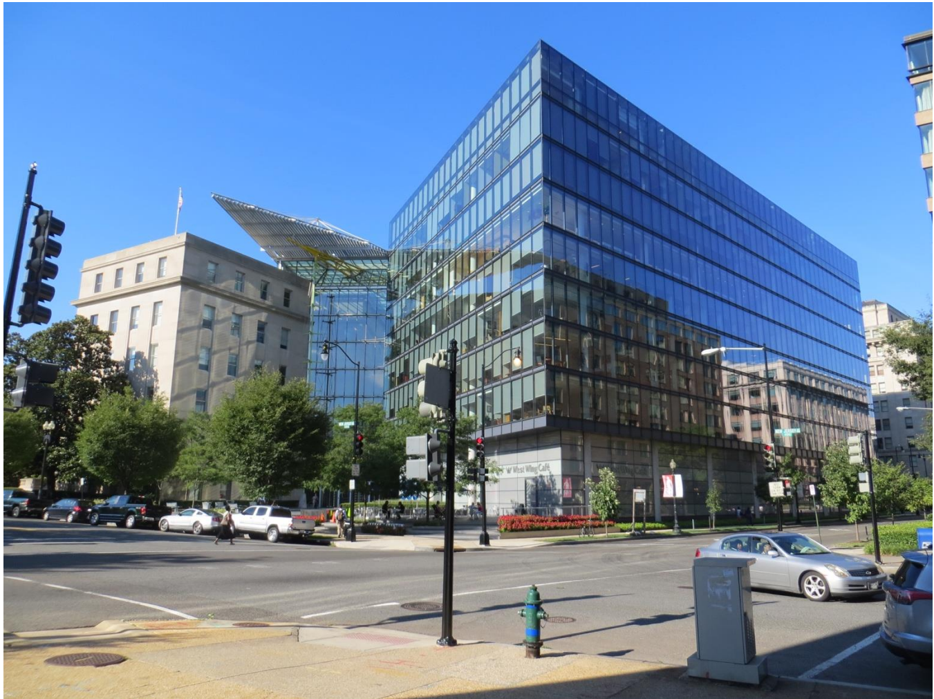
Illustration 5: View from northeast, showing 2009 addition. (John DeFerrari).
