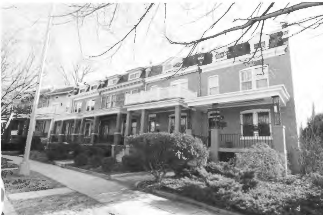
Photo 2 of 26: DC_Grant Circle Historic District_002.tif 4-7 Grant Circle, facing east
