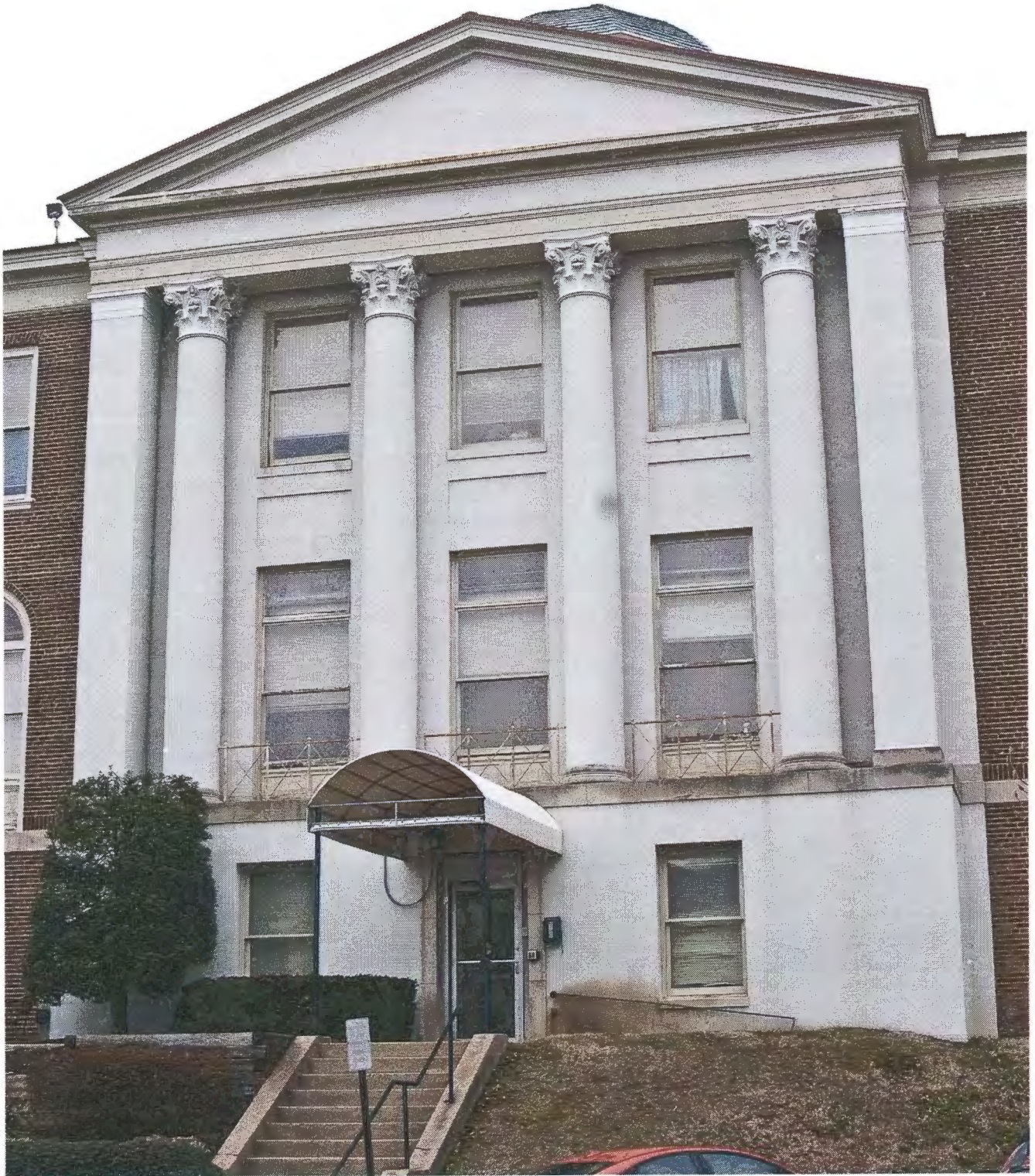
Image B6: Central Building, south facade portico, looking north.
