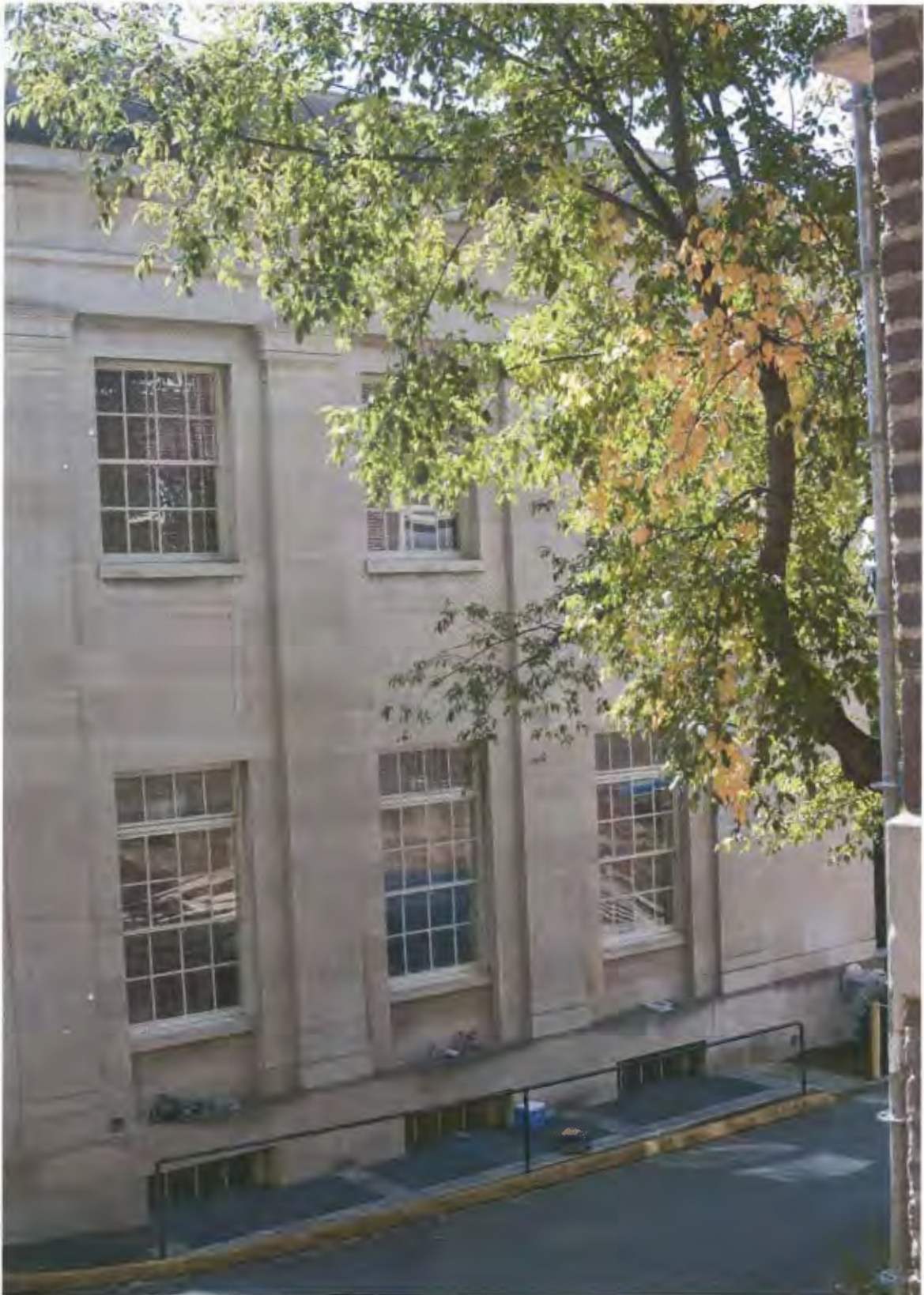
Image B12: Administration Building, north façade, looking SW.
