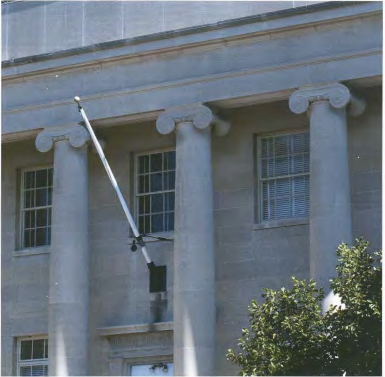
Image B11: Administration Building, detail of portico, west façade.
