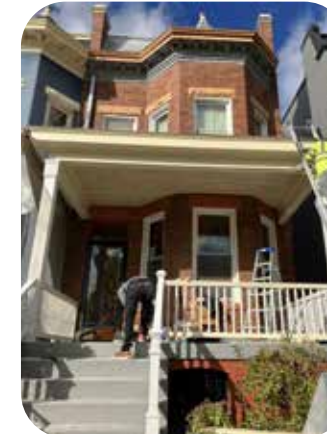
GRANT-SUPPORTED HOME REPAIR IN BLOOMINGDALE
