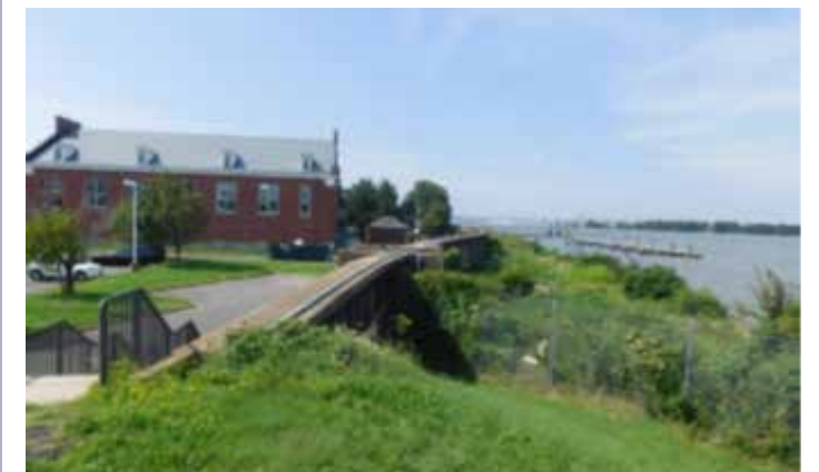
ANACOSTIA NAVAL AIR STATION SEAWALLS
