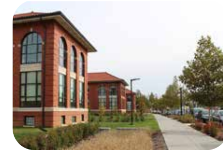
SAINT ELIZABETHS HOUSING AND STREETScape
