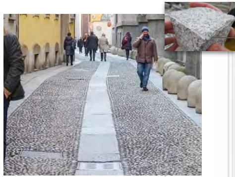
Cobble + Granite Pavers in Corso
