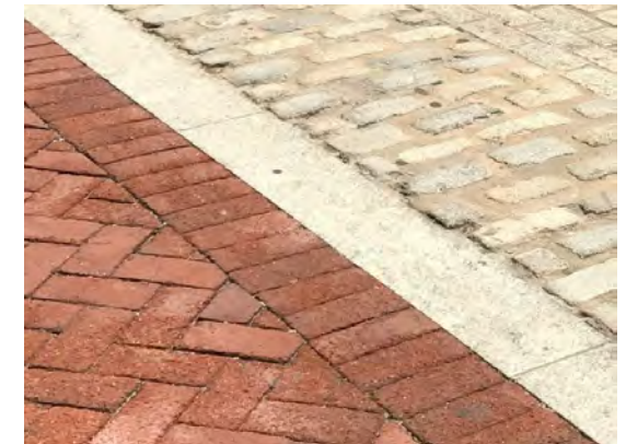
Brick Sidewalk w/ Granite Curb and Brick Gutter
