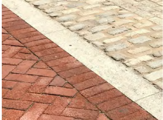
Brick Sidewalk w/ Granite Curb and Brick Gutter
