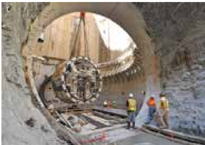
A H Street streetcar B 15th Street Cycle Track C Lady Bird boring machine creating new sewer tunnel to mitigate overflows
