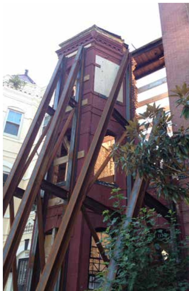
117 NEW YORK AVENUE NW SHOWING FACADE COLLAPSE AND STABILIZATION
